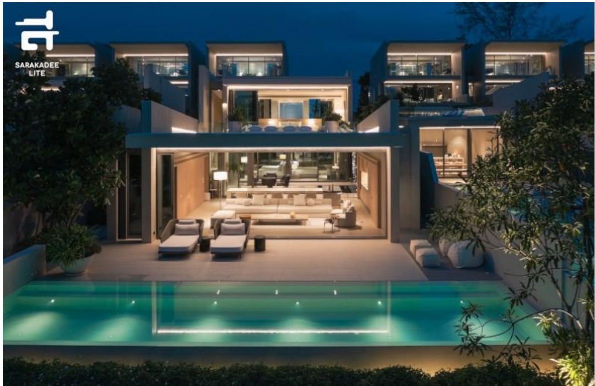
Veyla Natai Residences is a villa project spanning 5.8 Rai along Natai Beach, Tambon Khok Kloi, Phang Nga Province. It consists of 7 Beach Villas, each with 3 floors, located right on the beach, and 8 Sea Villas situated further inland. Among these, there are both private vacation homes and rental properties available for travelers who seek true privacy. The guest experience is managed and overseen by Elite Havens.
